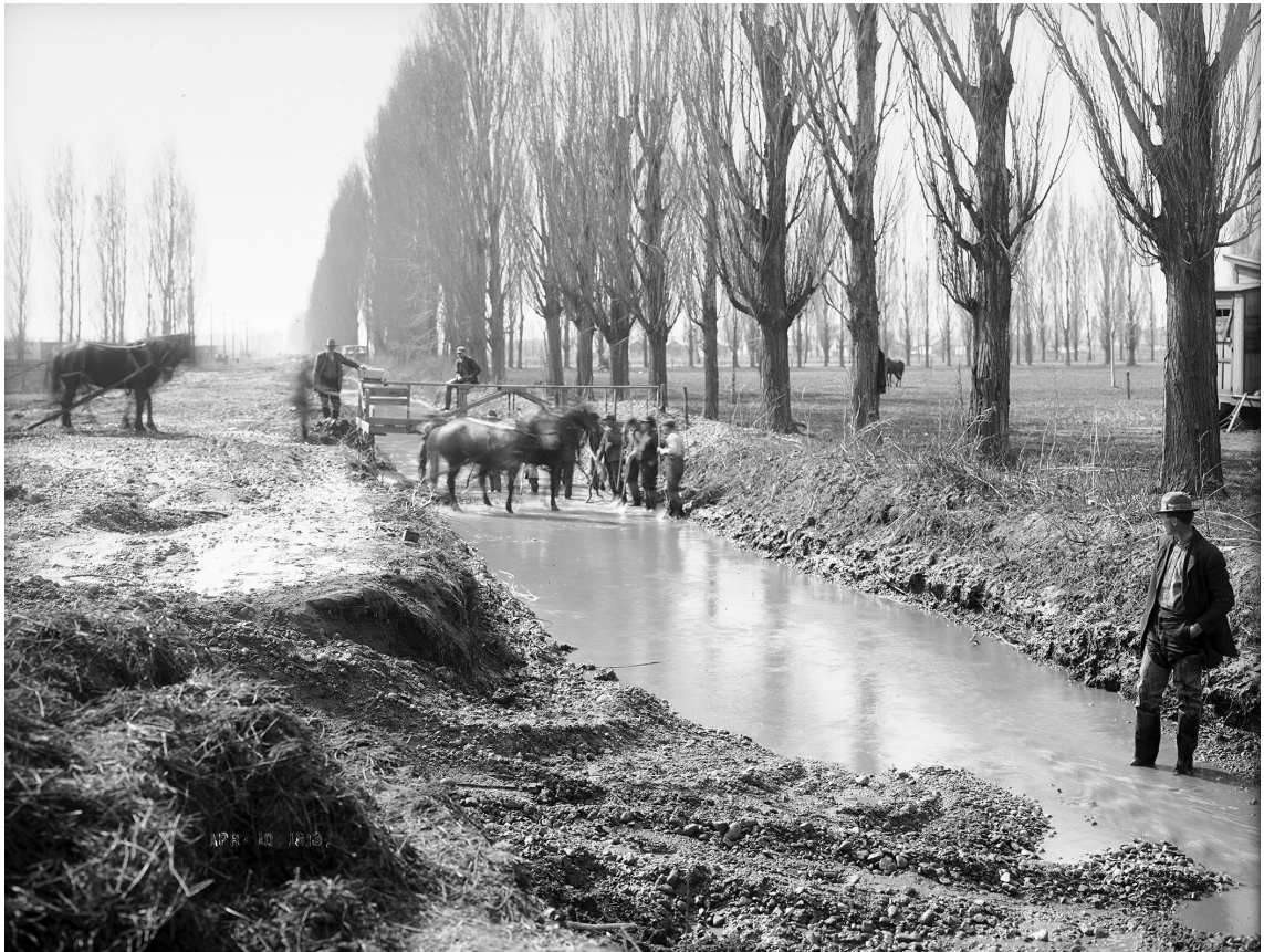
Workers dredge a canal in Salt Lake City in order to deepen the waterway in 1913. Utah Historical Society, city engineers no. 01594.
