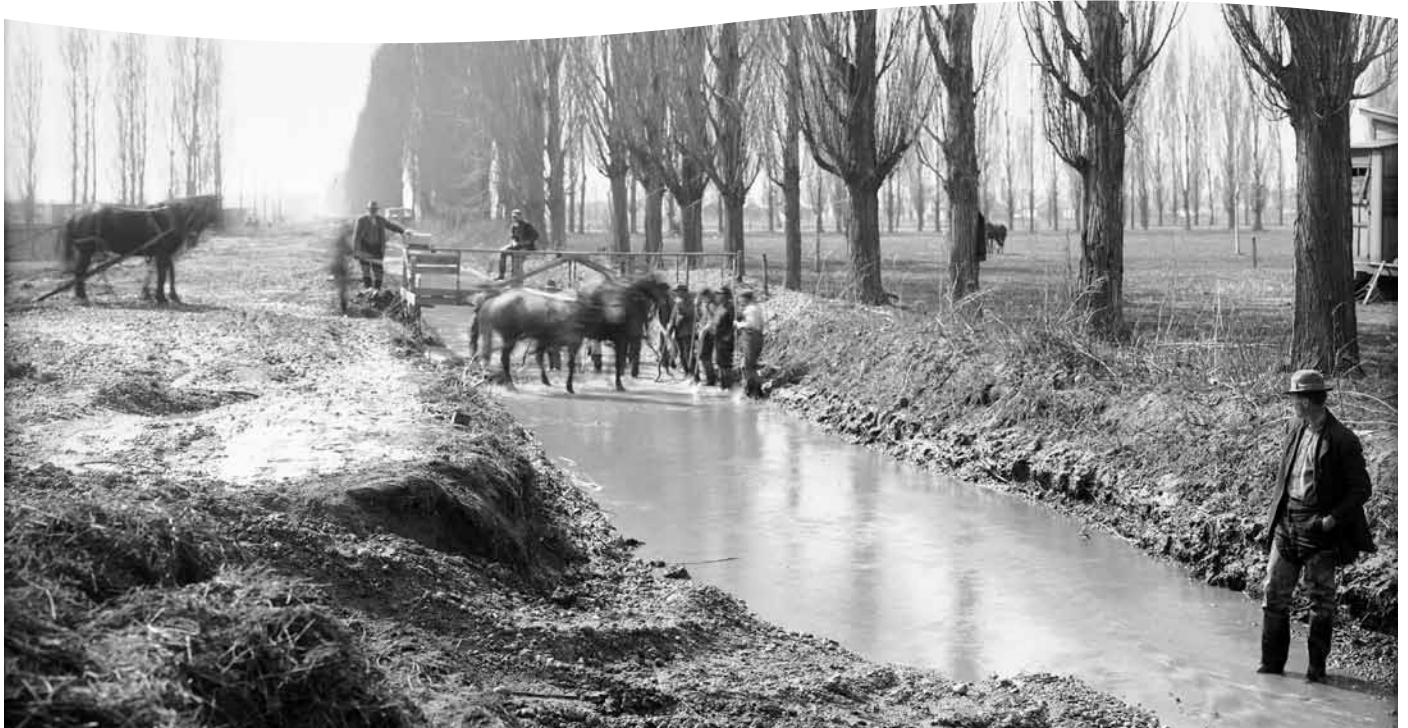
1000 South Canal, Salt Lake City, 1913. Such canals were common in early Salt Lake City. The poplar trees stabilized the banks as farmers manually dredged deeper to encourage water to spread through the settlement. Utah State Historical Society.
