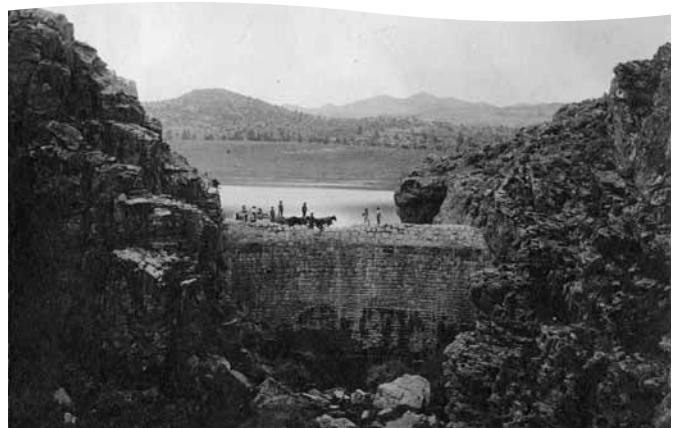
Enterprise Dam, Washington County, c1910. Water catchment in flood-prone southern Utah developed as a way to regulate extremes in the flow of water, as well as use rights. Utah State Historical Society.
