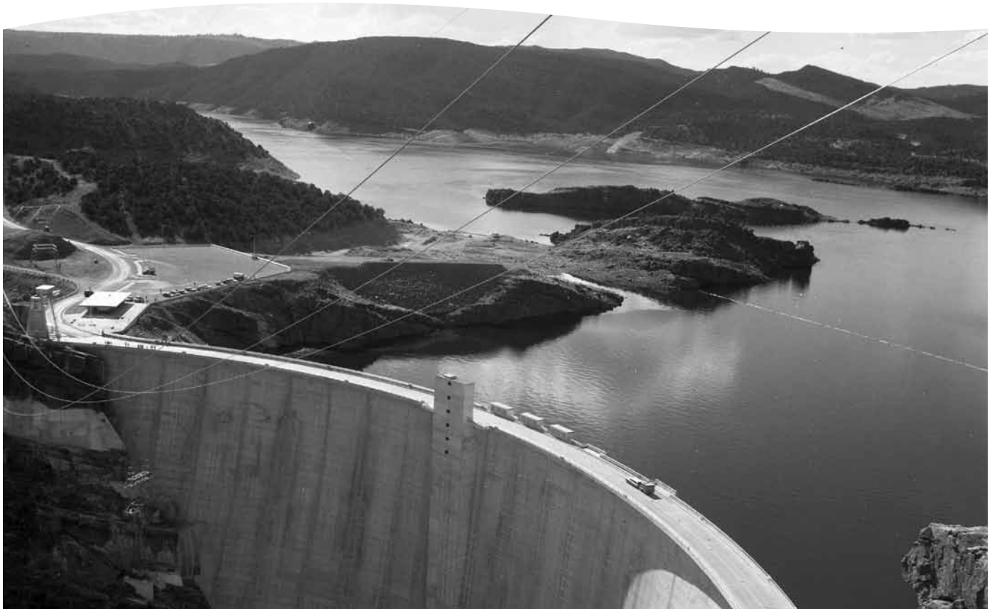
Flaming Gorge Dam, 1964. The construction of Flaming Gorge Dam on the Green River was met with resistance, and opinions over the finished product were mixed. By the time construction wrapped up in 1964, it wore a price tag of 65 million dollars. Uintah County Library Regional History Center.
