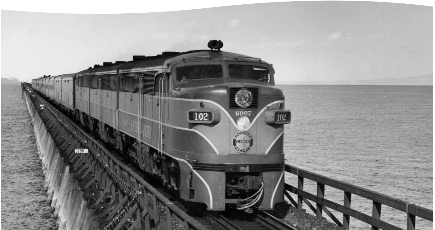
Southern Pacific Train, Lucin Cutoff, c1959. A causeway across the lake replaced the aging wooden trestle, separating the lake's waters into north and south arms and causing vastly different saline levels. Utah State Historical Society.
