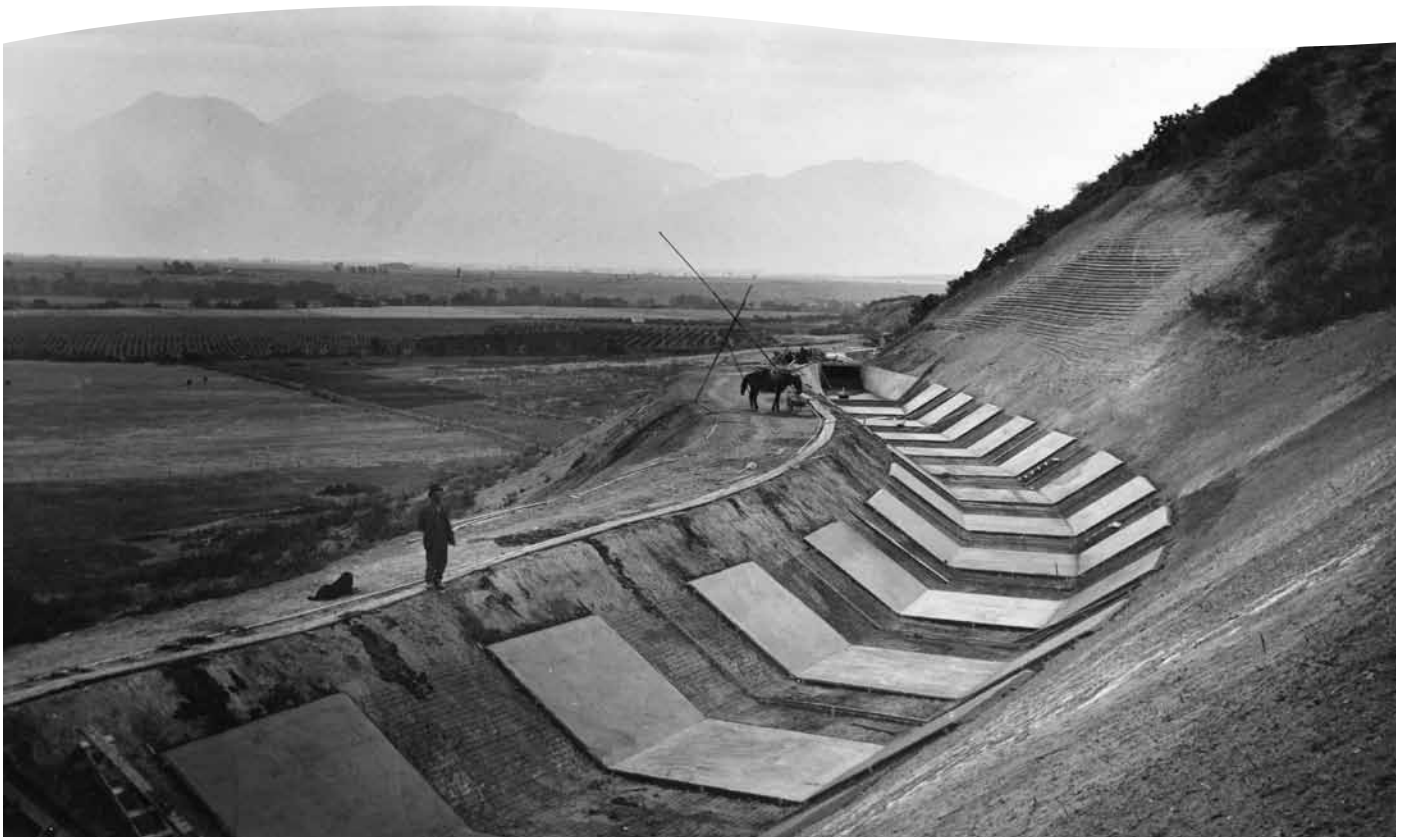
Construction of Strawberry Highline Canal, Salem, 1915. The Strawberry Valley Project was the first major inter-basin transfer of water in the state. Utah State Historical Society.
